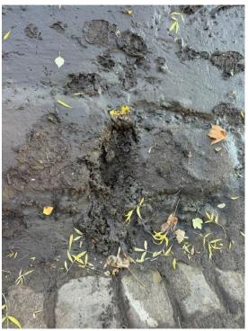
Concrete path covered in silt. The concret is broken up and easily displaced when aggetated by foot.
