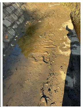
Build-up of silt on top of concrete path.
