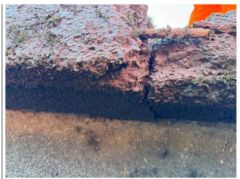
Large section loss in capping beam with exposed steel reinforcement. Crack through the width of the capping beam.
