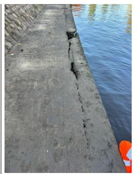
Failed capping beam, no longer sufficiently supported and breaking away from the concrete path. Large cracking, exposed and deformed steel reinforcement in capping beam.
