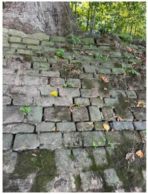
Missing mortor between stones on the pitched stone embankment.
