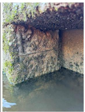
83 Concrete spalled and exposed steel reinforcement at the top of the pile.
