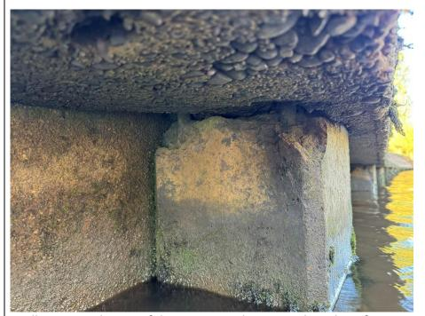
Spalling on on the top of the concrete pile, exposed steel reinfocement.
