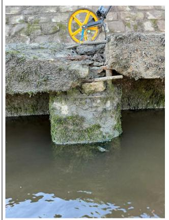
Spalled and loose concrete on top of the capping beam and pile, with corroded and deformed steel exposed.
