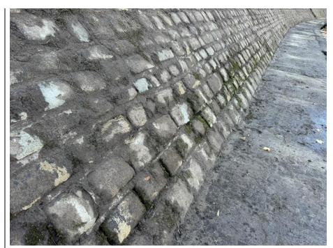
Missing mortar on pitched stone embankment.
