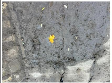
Build-up of silt on top of the concrete path. Large crack in the slab propagating from the capping beam to the bottom of the pitched stone.
