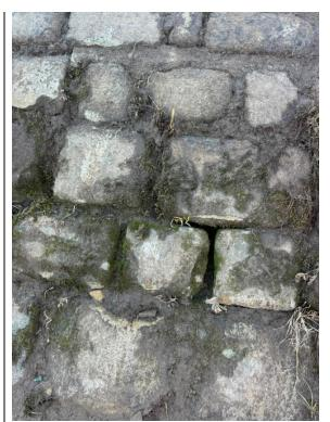
129 Missing mortar on pitched stone embankment.
