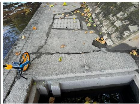
93 Cracking in the concrete path around manhole.
