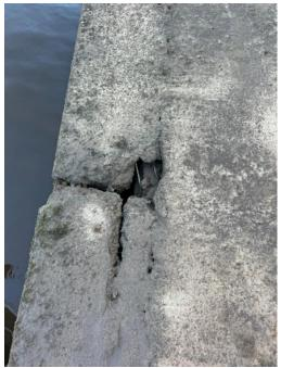
Cracking between two capping beams with exposed steel reinforcement over the pile support. Large gap between the capping beam and concrete path formed, can see the top of the retaining wall.
