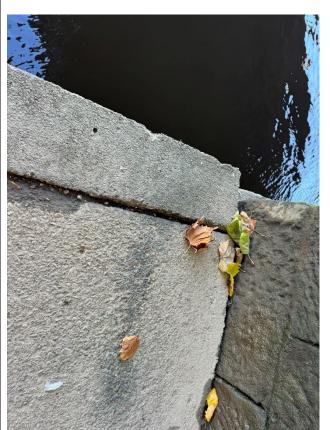
Gap between the concrete path and capping beam. End of the path, Scarborough Rail Bridge masonry visible.
