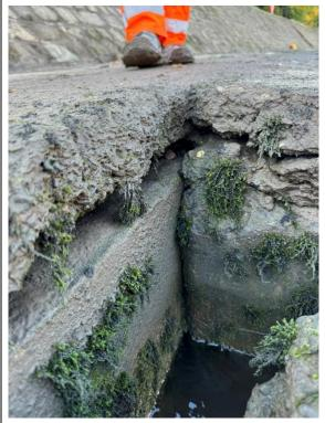
Gap between the concrete path and top of the retaining wall.
