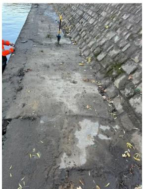
27 Cracks in the slab and various patches of slab construction.
