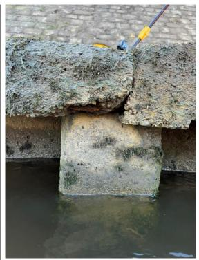
Spalling of concrete to the underside of the capping beam. Corroded steel reinforcement is exposed.
