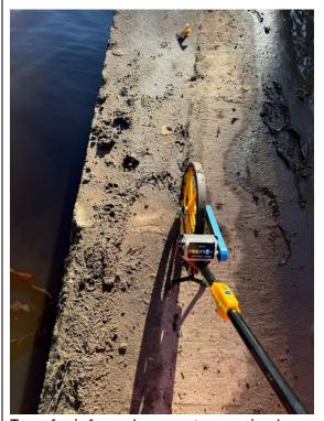
Top of reinforced concrete capping beam and concrete path.
