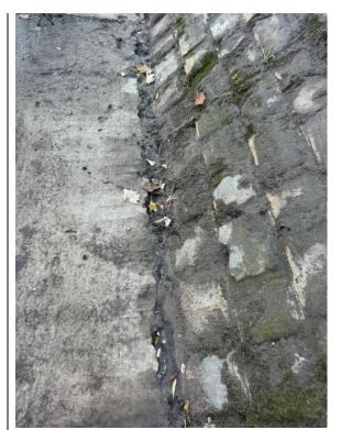
Void in concrete slab at the base of the pitched stone.
