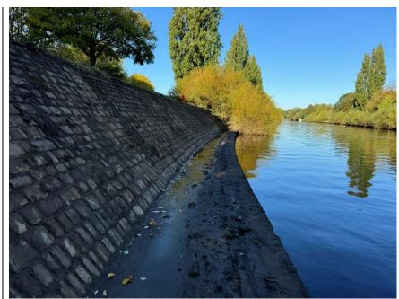
View from the concrete path looking westwards, away from the Scarbourough Rail Bridge. Silt build-up and water pooling on the path.
