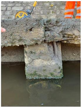
Concrete spalling on the side of the concrete capping beam and top of the pile. Spalling has exposed the steel reinforcement. The reinforcemet is corroded.
