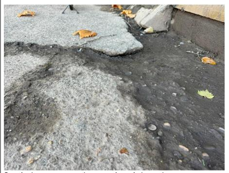
Step in the concrete path, corner is a trip hazard.
