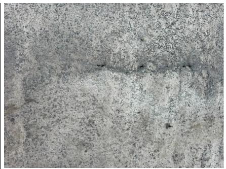
77 Small crack forming on the concrete path.
