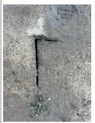
Gap between the concrete path and capping beam. Step in the path.
