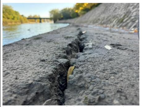
Large crack between the capping beam and concrete path.
