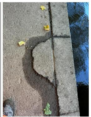
Minor spalling on the surface of the concrete path.
