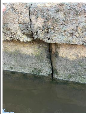
Crack down the capping beam and down the retaining wall.
