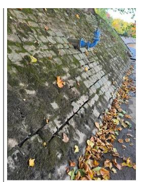
101 Missing mortor between stones on the pitched stone embankment.
