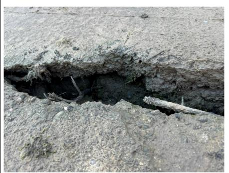
Large gap between the capping beam and concrete path. Exposed steel reinforcement.
