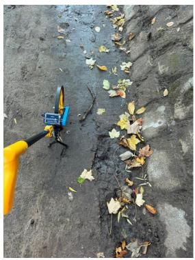
Void and broken up concrete slab at the base of the pitched stone. Areas of loose concrete at the surface.
