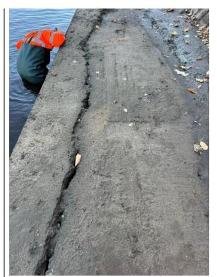
Large crack between the capping beam and concrete path.
