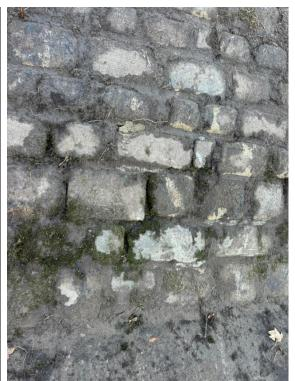
Missing mortar on pitched stone embankment.
