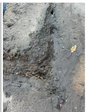
Loose concrete aggregate on top of the capping beam.
