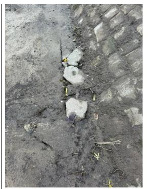
Void and broken up concrete slab at the base of the pitched stone. Areas of loose concrete at the surface.
