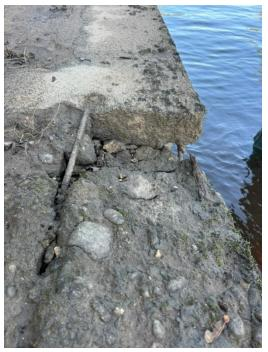
Loss of section on the capping beam, concrete spalled and broken away exposing deformed steel reinforcement.
