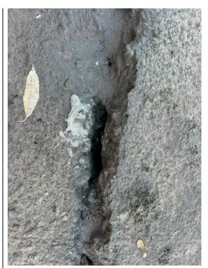
37 Large crack between the capping beam and concrete path.
