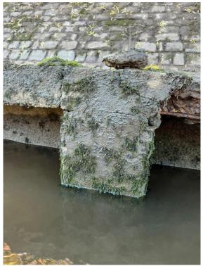
Concrete spalling and exposed corroded steel reinforcement in the capping beam. Surface cracks on the pile.
