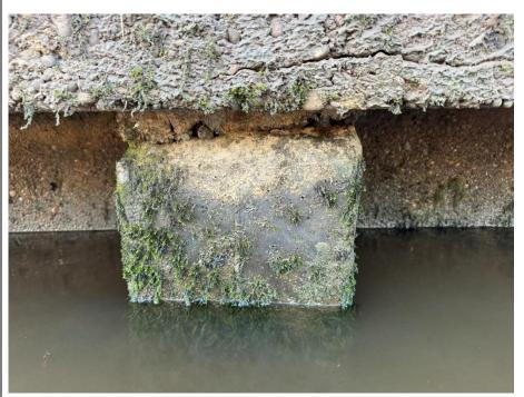
Close up of concrete spalling at the top of the pile with exposed corroded steel reinforcement.
