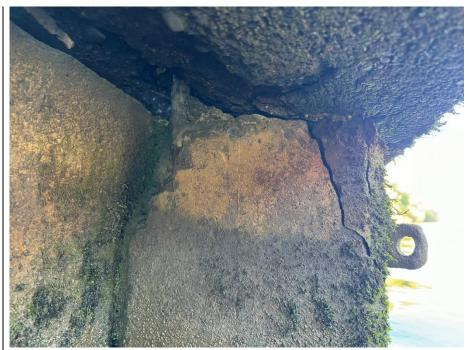
Spalling of concrete at the top of the pile. Steel reinforcement bars are exposed.
