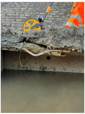
Severe cracking in the capping beam, with concret spalling. Exposed, deformed and corroded steel reinforcement.
