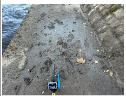
Build-up of silt on top of the concrete path.
