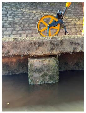
Gap between the capping beam and pile. The capping beam not bearing onto the pile. Steel reinforcement exposed on the top of the pile.
