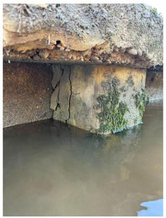
Spalling at the back of the pile and underside of the capping beam.
