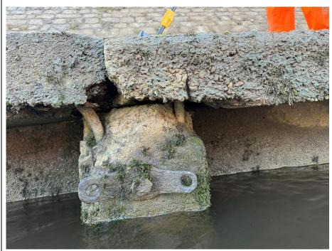
Spalling of concrete at the top of the pile and underside of the capping beam. Corroded steel reinforcement bars are deformed and exposed.
