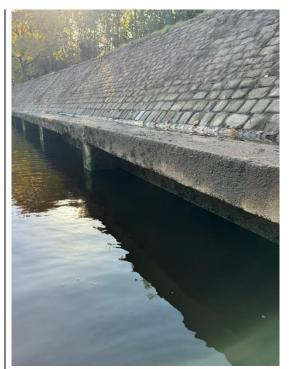
Photo of capping beam in ok condition.
