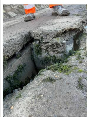
Failed capping beam, no longer sufficiently supported and breaking away from concrete path. Large cracking and deformed steel reinforcement exposed in the capping beam and pile.
