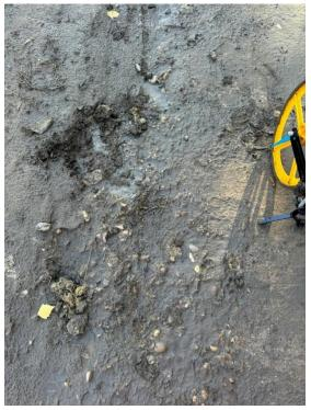
Loose aggregate on concret slab surface.
