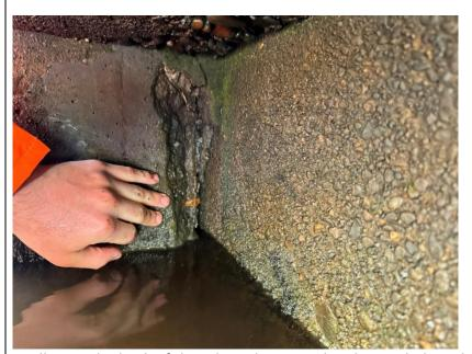
Spalling at the back of the pile with exposed and corroded steel reinforcement.
