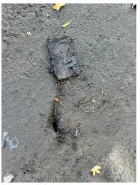
Small gap in joint between the concrete path and capping beam.
