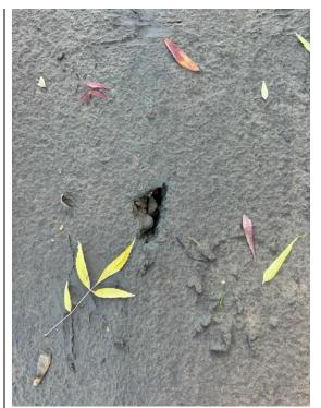
Small gap in joint between the concrete path and capping beam.
