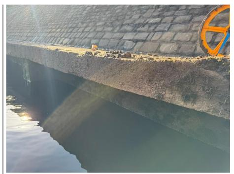
Photo of capping beam in ok condition.
