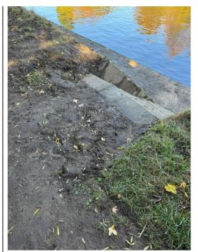
Top of embankment steps. The top steps are out of place.
