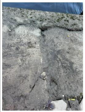
Crack between the concrete path and capping beam. Broken up concrete slab at the base of the pitched stone retainig wall. Areas of loose concrete at the surface.
