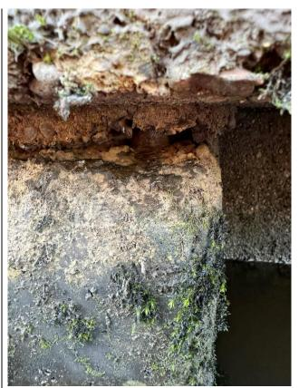
25 Close up of concrete spalling at the top of the pile with exposed corroded steel reinforcement.
