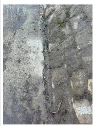
Gap forming between the pitched stone and concrete path.
