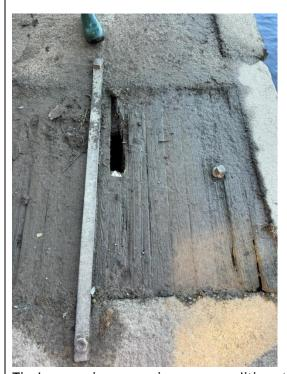
Timber service cover in poor condition, timber is rotting.
