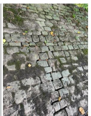
103 Missing mortor between stones on the pitched stone embankment.
