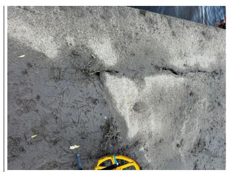
63 Crack between the capping beam and concrete path.
