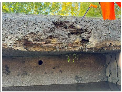
Concrete spalling and exposed corroded steel reinforcement on the capping beam. Cracking to the rear of the pile.
