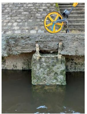
Spalled concrete on the side of the capping beam and top of the pile.
