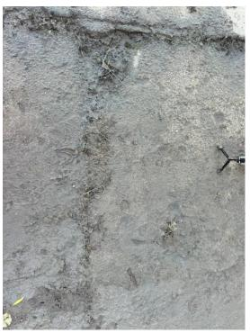
Crack in the concrete path, propogating from the capping beam to the pitched stone.
