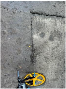
Gap between the concrete slab and capping beams. Gap between two slabs.
