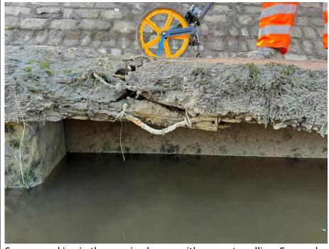
Severe cracking in the capping beam, with concret spalling. Exposed, deformed and corroded steel reinforcement.
