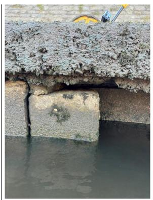
Large gap between the top of the pile and capping beam. Aggregate visible at the surface of the capping beam. Start of the retaining wall to the left of the pile.
