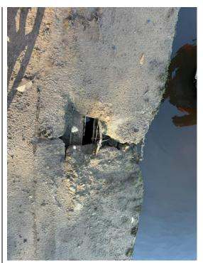
Loss of section on the capping beam, concrete spalled and broken away exposing deformed steel reinforcement. Can see through the capping beam to the top of the pile underneath.
