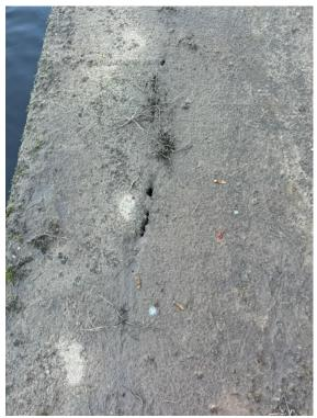
Gap forming between the concrete path and capping beam.
