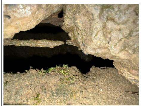
Top of retaining wall is visible through the capping beam. There is a void behind the retaining wall.
