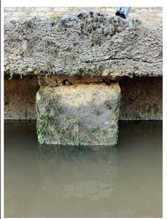
Cracking in the side of the capping beam. Concrete spalling at the top of the pile with exposed corroded steel reinforcement.
