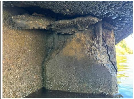
Cracking at the top of the pile. Spalling on on the top of the concrete pile, exposed steel reinfocement.
