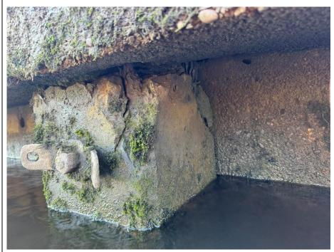
Spalling of concrete at the top of the pile. Corroded steel reinforcement bars are exposed.
