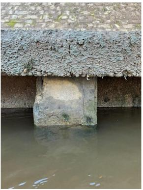
Cracking at the top of the pile. Spalling on on the top of the concrete pile, exposed steel reinfocement.
