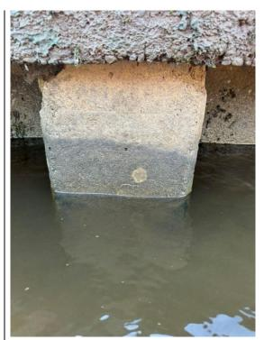
63 Minor spalling to top corners of the pile.
