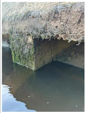
Aggregate visible at the surface of the capping beam. Crack at the back of the pile.
