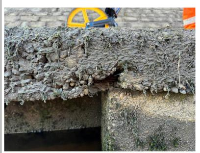
Spalled concrete under the capping beam with exposed and corroded steel reinforcement.
