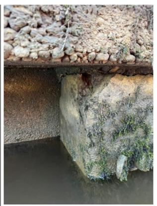
Spalling on on the top of the concrete pile, exposed steel reinfocement.
