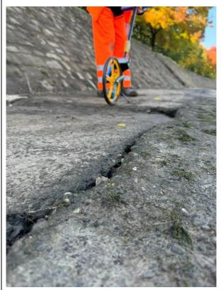
Crack between the concrete path and capping beam.
