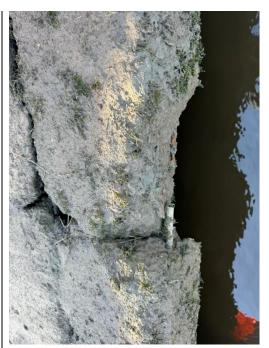
Cracking between two capping beams with exposed steel reinforcement over the pile support. Gap between the capping beam and concrete path formed.
