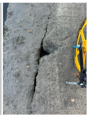
Gap between the concrete path and capping beam.
