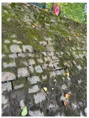
Missing mortor between stones on the pitched stone embankment.
