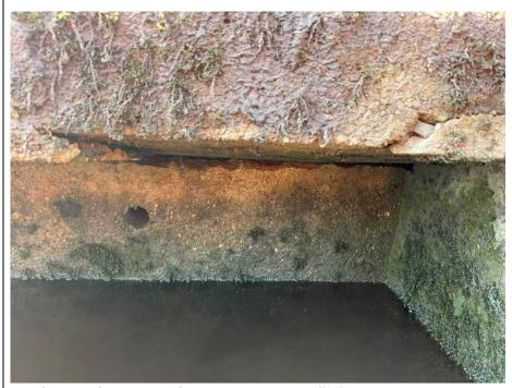
Cracking in the capping beam. Retaining wall okay.
