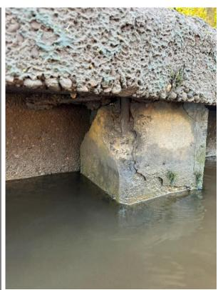
Cracking at the top of the pile. Spalling on on the top of the concrete pile, exposed steel reinfocement.
