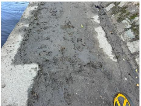
Top of the concrete path coverd in silt.
