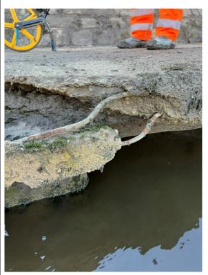
Deformed steel reinforcement in the capping beam at point of failure.
