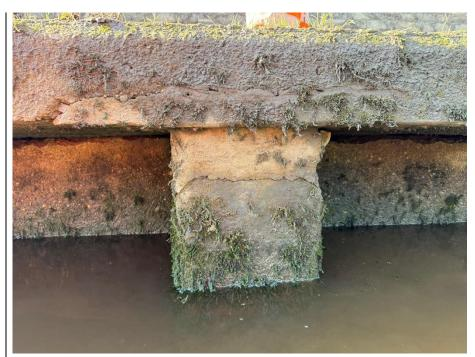
Cracking at the top of the pile and side of the capping beam. Retaining wall is ok.
