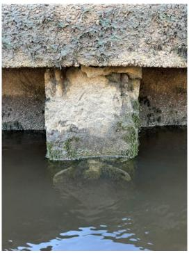
Spalling of concrete at the top of the pile. Steel reinforcement bars are exposed.
