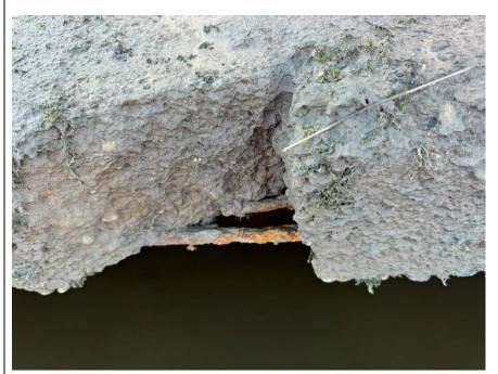
Spalled concrete with exposed corroded steel reinforcement on the capping beam.
