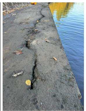
Large crack between the capping beam and concrete path. The capping beam is tilting towards the river, braking away from the concrete path.
