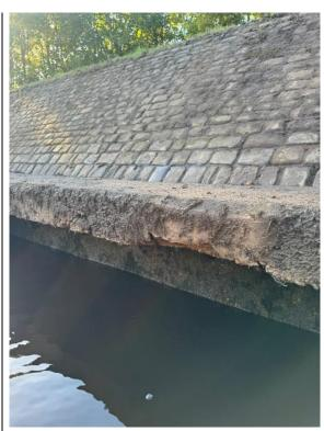
Photo of concrete spalling on the bottom of the capping beam.
