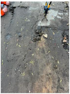
Cracks in the slab and various patches of slab construction.
