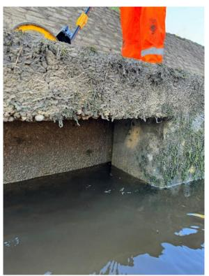
Aggregate visible at the surface of the capping beam. Gap between the retainig wall and pile.
