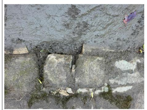
Missing mortar on pitched stone embankment.
