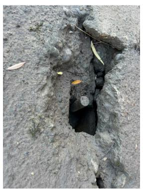
Exposed pile steel reinforcement, protruding through gap in capping beam and concrete path.
