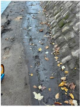
Build up of silt on the concrete path.
