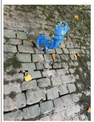
Missing mortor between stones on the pitched stone embankment around a service valve.
