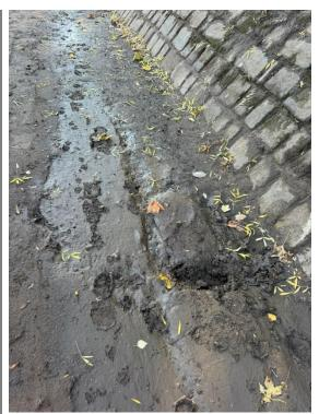
Concrete path covered in silt. The concret is broken up and easily displaced when aggetated by foot.
