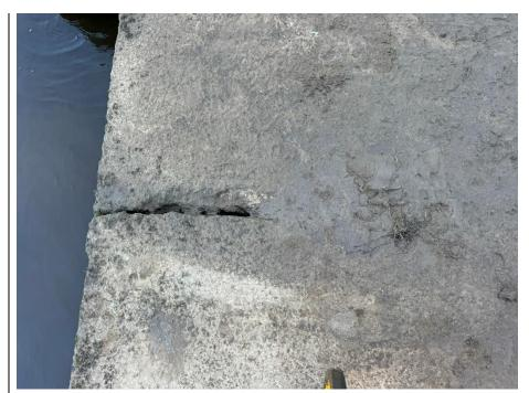
79 Crack in the concrete capping beam.
