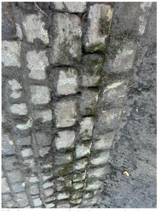
Missing mortar on pitched stone embankment.
