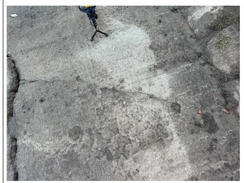
Crack between the capping beam and concrete path.
