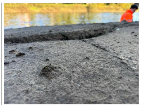
Crack between the capping beam and concrete path. The capping beam is moving away from the concrete path.
