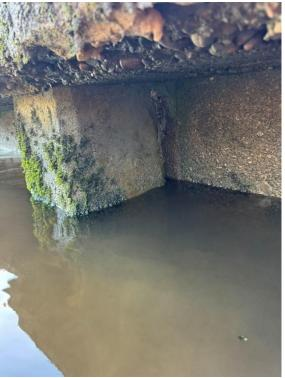
Aggregate visible at the surface of the capping beam. Spalling at the back of the pile with exposed and corroded steel reinforcement.
