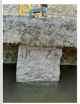
Spalled concrete at the top of the pile, with corroded steel reinforcement exposed.
