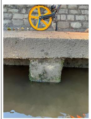
Photo of capping beam in ok condition. Cracks in the top of the pile.
