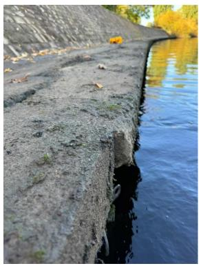
Large crack between the capping beam and concrete path. The capping beam is tilting towards the river, braking away from the concrete path.
