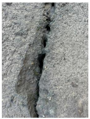
Large crack between the capping beam and concrete path.
