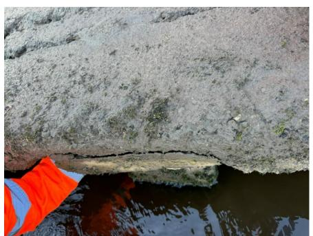
Cracking and loose concrete on the side of the capping beam above the pile.
