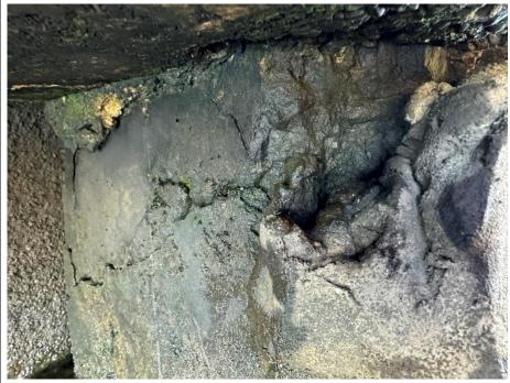
Spalling of concrete at the top of the pile.
