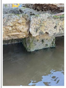
Failed capping beam, no longer sufficiently supported and breaking away from concrete path. Large cracking and deformed steel reinforcement exposed in the capping beam and pile.
